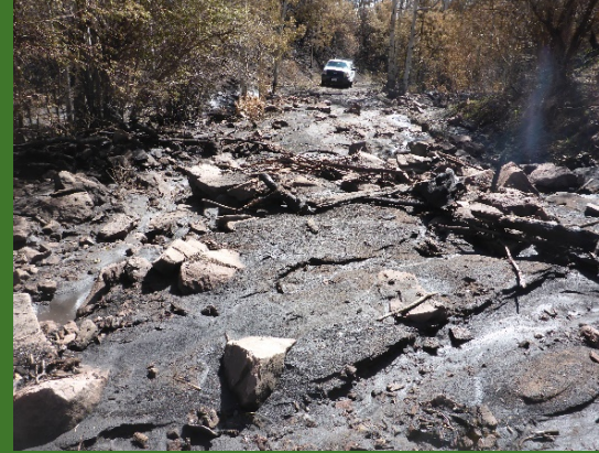
Private road washed out by debris flow
