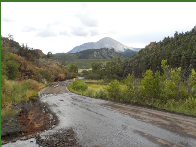
0.7 inches of rain produced these overtopping flows of CO Hwy 12
