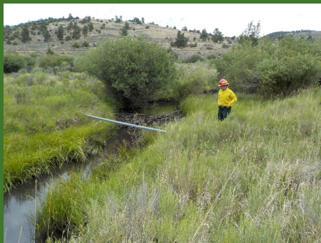
Buried utility line exposed at crossing of Wagon Creek within Forbes Park
